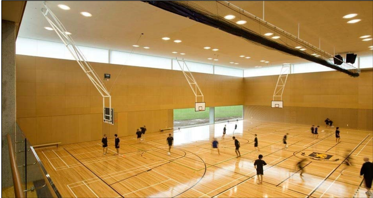
Figure 26: Auckland Grammar School gym sports centre. High level translucent glazing with sloped ceiling to minimise glare. Limited low level windows for view; glare risk mitigated by non-reflective external surface.
