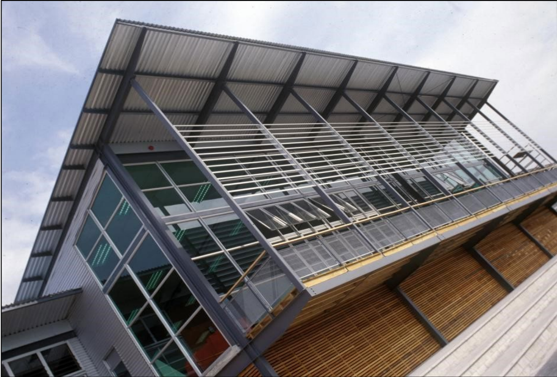
Figure 16: Combination of sunscreens and overhangs provide a good level of solar shading and daylighting
