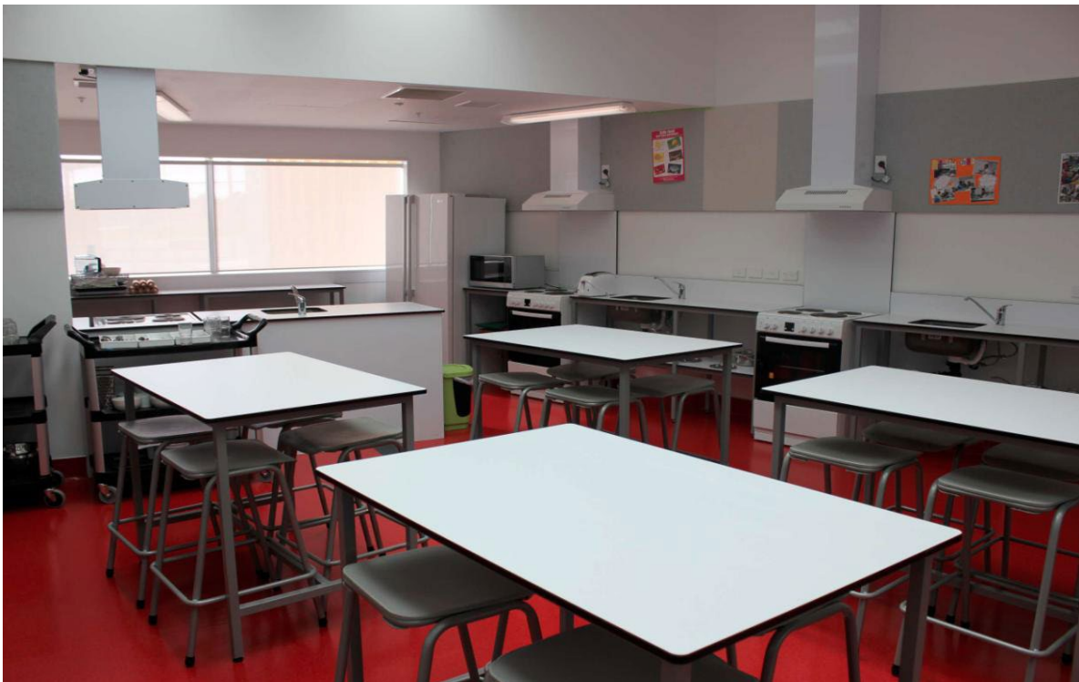
Figure 20: A secondary school food technology space with residential grade cookers and residential extraction
