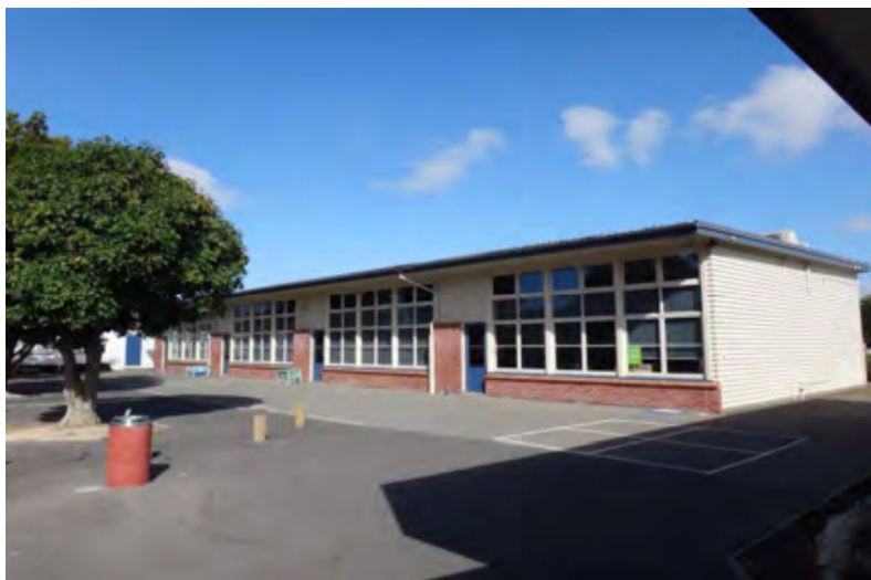
Figure 12: Canterbury Block reference design - an example of existing infrastructure with a high WWR
