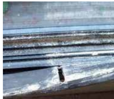
Chalking on aluminium joinery.
