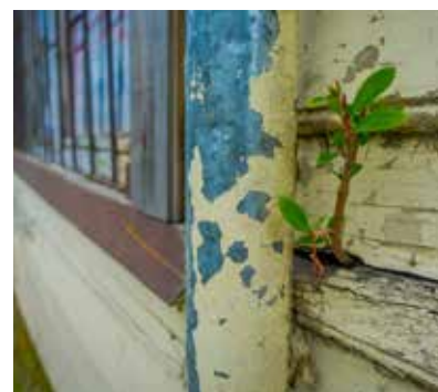
Plant growing in wall cladding.
