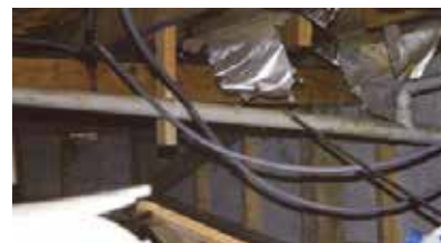
Loose wiring.
