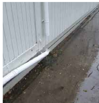
Disconnected downpipe.
