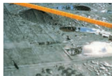
Bubbles appearing under membrane.
