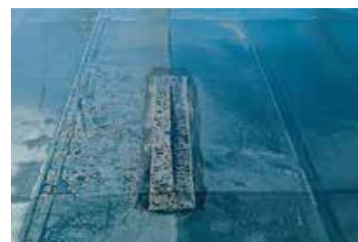
Patch repair to joint.
