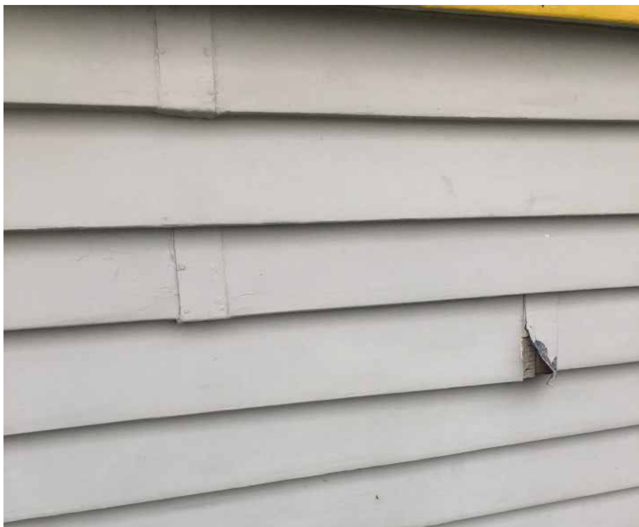
Repair soaker flashing at weatherboard junction.
