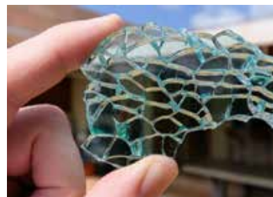
Broken toughened safety glass.
