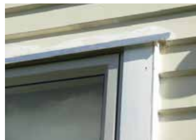
Aluminium window retrofitted into existing wall with new head flashing, boxed trim and scribe.
