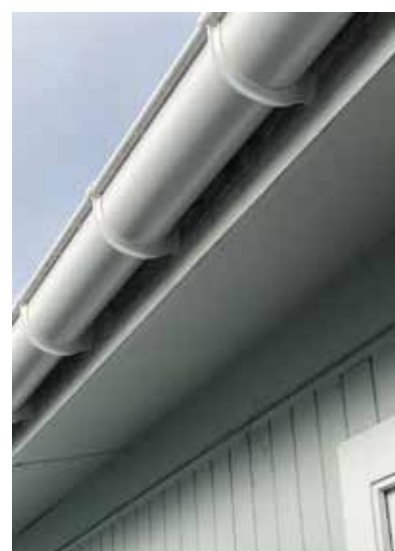
Gutter in good condition.
