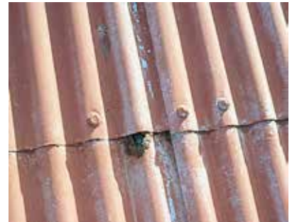
Damaged sheets.
