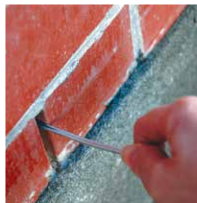
Cleaning drainage slots at bottom of veneer to allow for drainage of cavity.
