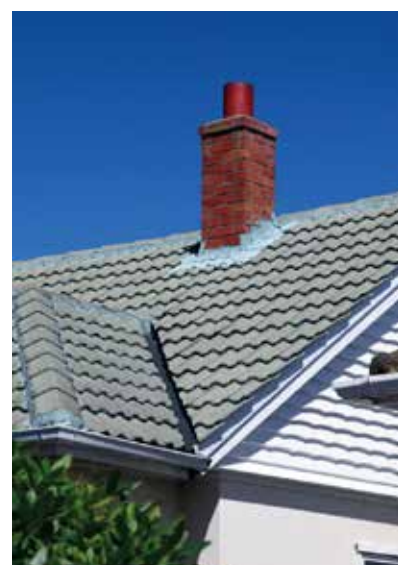
Heavyweight roof (concrete tiles).
