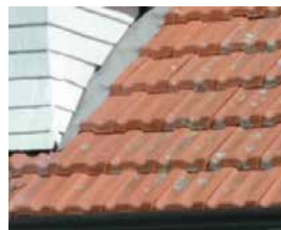
Lead flashing to clay tiles.
