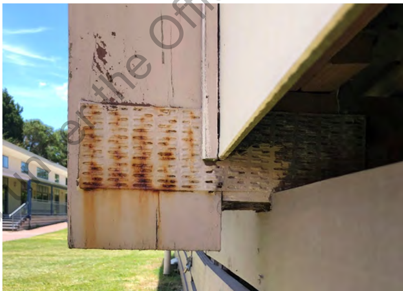
Figure 7: Portal leg-bearer connection - R Block
